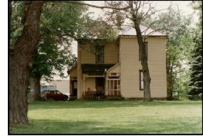
George Foulke Farm House
