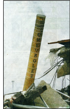
2008, Smokestack coming down
