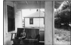
c. 1947, Walt Jr - Front Porch - 16th St house
